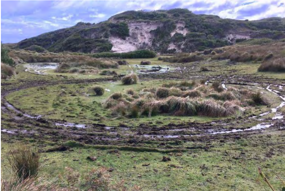
FIGURE 2.2. DAMAGE AT ARTHUR-PIEMAN CONSERVATION AREA CAUSED BY 4WD VEHICLES. SOURCE: CRAIG BROADFIELD 90
